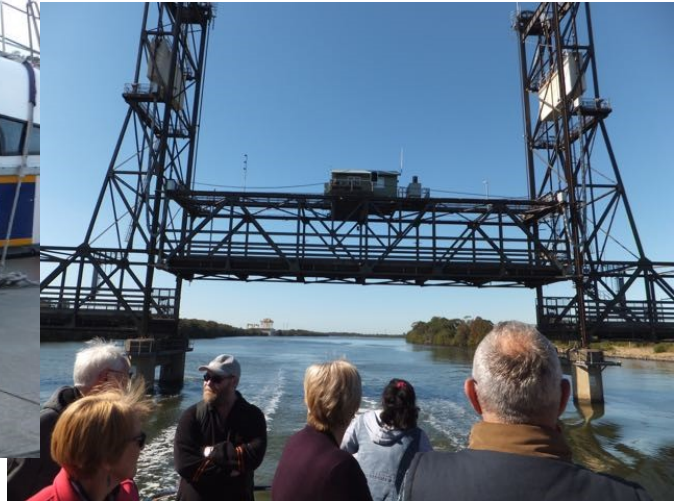
Under the raised Hexham Bridge
